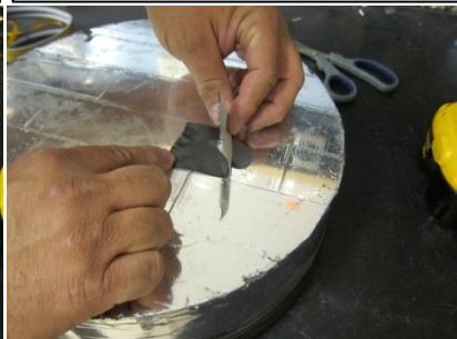
Fig. 23. Septa held in place with tape.
