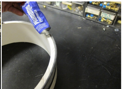
Fig. 9. Thin layer of contact cement applied to PVC edge.
